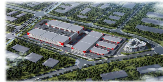
Self-built Sorting Center in Guangzhou As-built renderings (Expected to be put into use in 2025)
